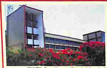
SMJV, Sandhurst Road, Mumbai
